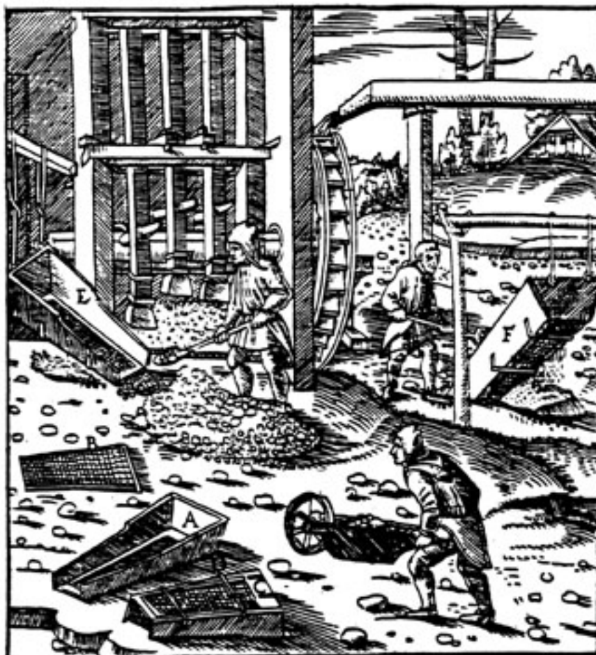
Drop hammers driven by overshot water-wheel (after Agricola, c. 1556)
